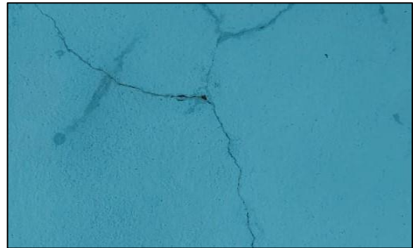
Fig.8 Diagonal Cracks
