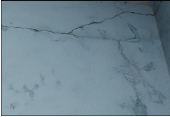
Fig.4 Shear Crack
