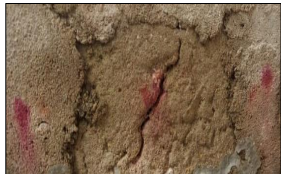
Fig.9 Masonry Cracks
